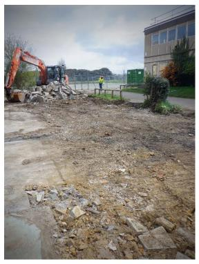
Plate 2. Removing concrete surfaces (looking North)
