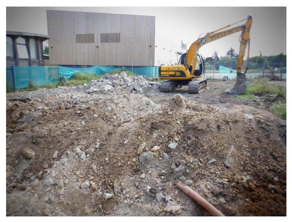
Plate 3. Removing foundation footing (looking NNW)
