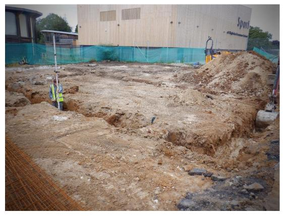
Plate 8. Foundation trenches (Looking NW)
