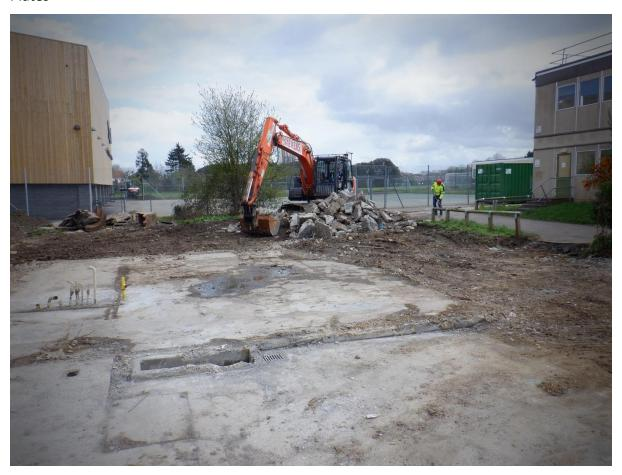
Plate 1. Removing concrete foundations and surfaces (looking North)
